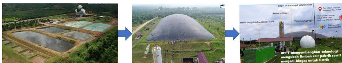
Figure 28 Schematic Illustration of POME Conversion to Biogas for Electricity Production 27
