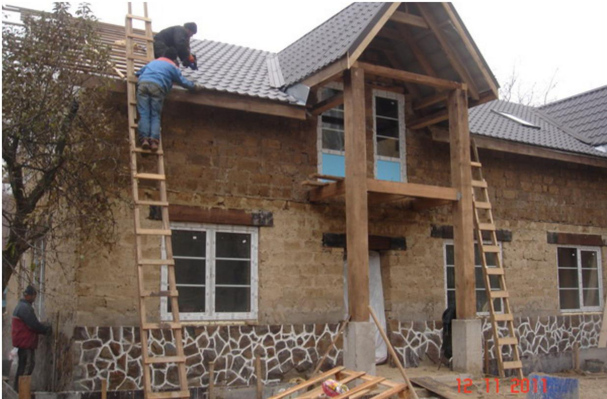
PICTURE 4. Construction of straw brick houses in Kyrgyzstan. Source: construction portal USTA ([www.usta.kg](http://www.usta.kg))
